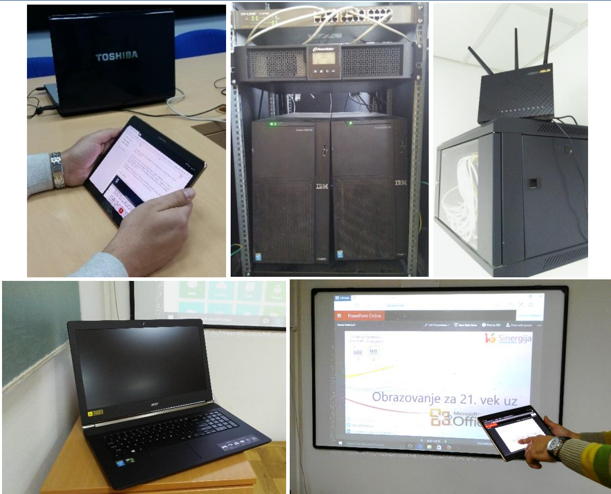
Picture 2. Equipment installed at University of Kragujevac
